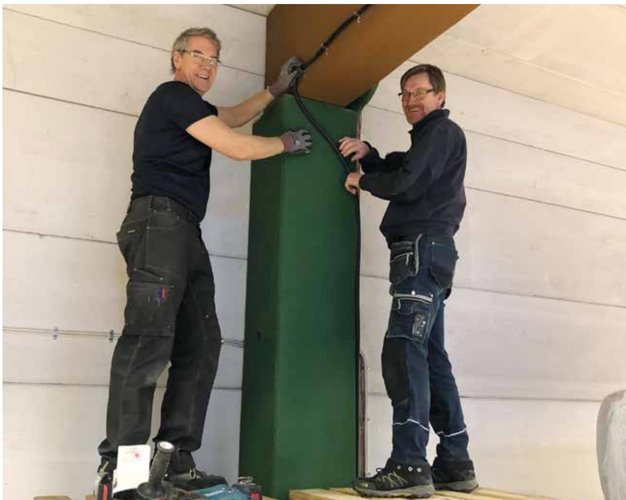
The storage area in the loft is completed. Leif, property manager, on the left in picture and Mats, technician, on the right.
